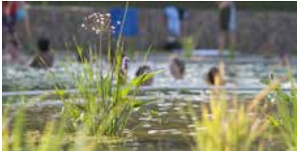
A submerged filter with gravel and plants under the water surface.
